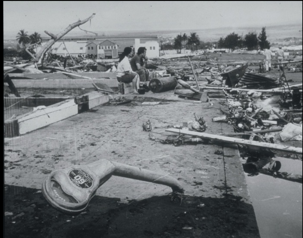
Tsunami damage in Hawaii
