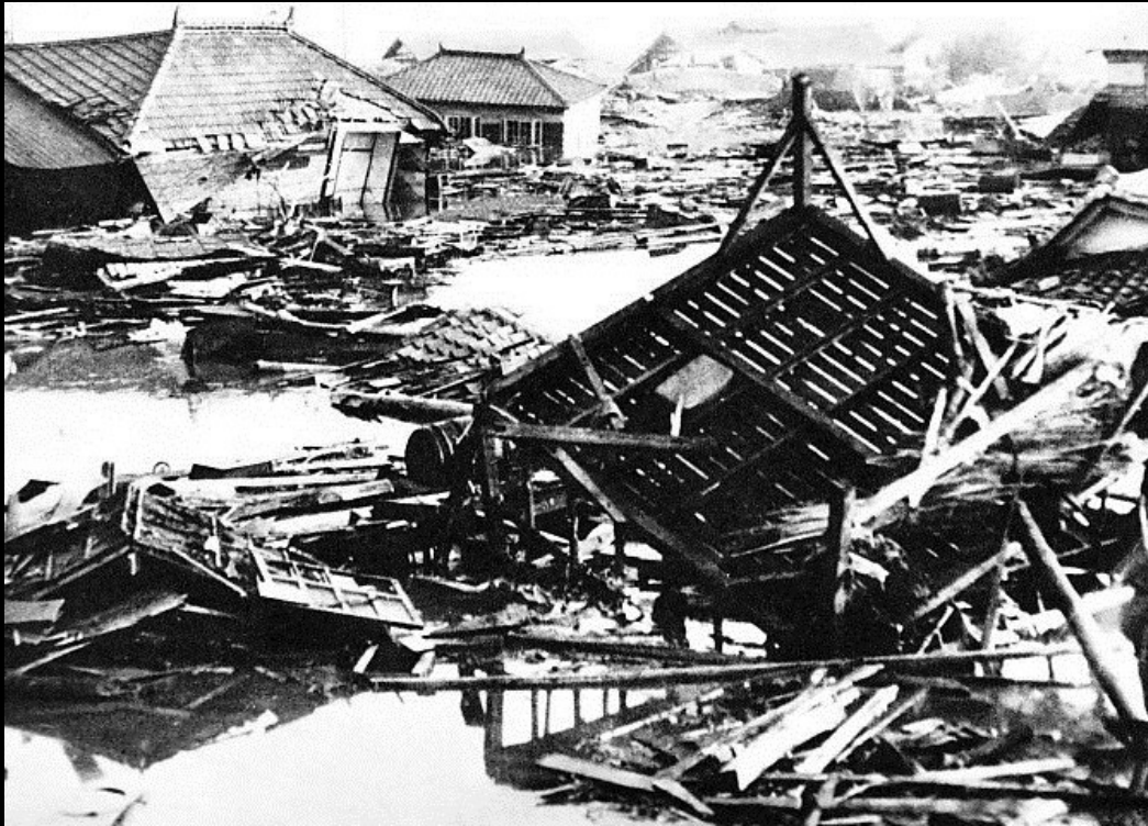
Tsunami damage in Japan
