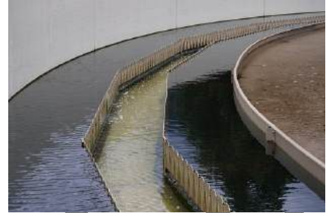
Sewage treatment facilities reduce water contamination.
