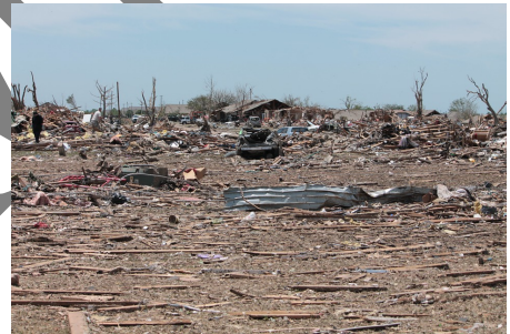
Tornado damage can be severe.
