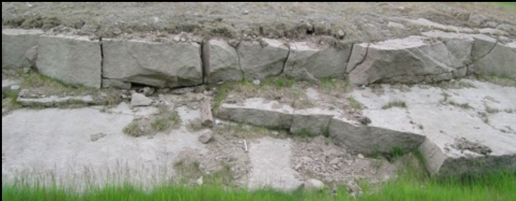
Pressure release in granite. Nannestad, Norway.
