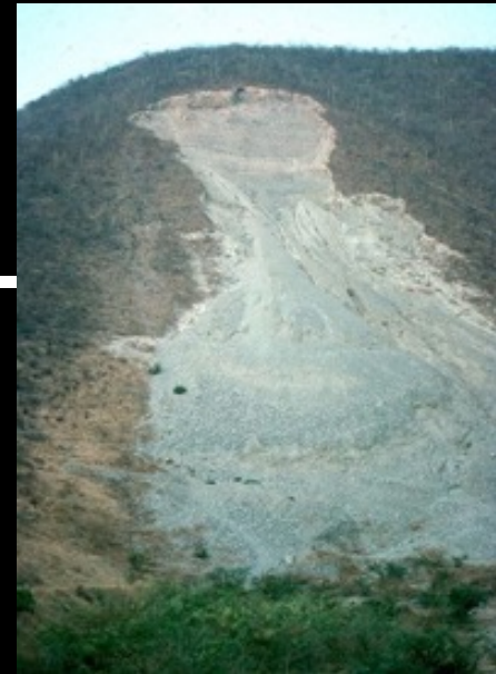
A rockslide in Guerrero, Mexico
