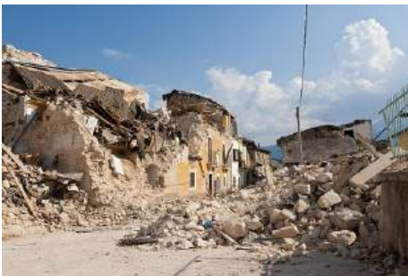
Earthquakes can destroy buildings.
